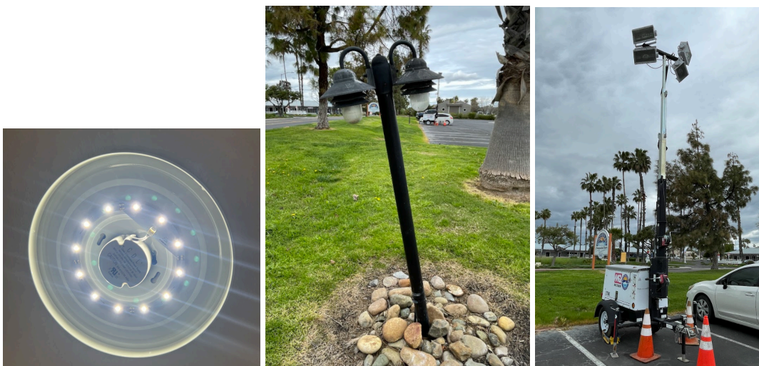
Figure 3.6: Existing Lighting (Community Center)
